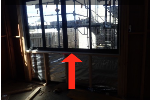
No packers between sill and sill trimmer plate
